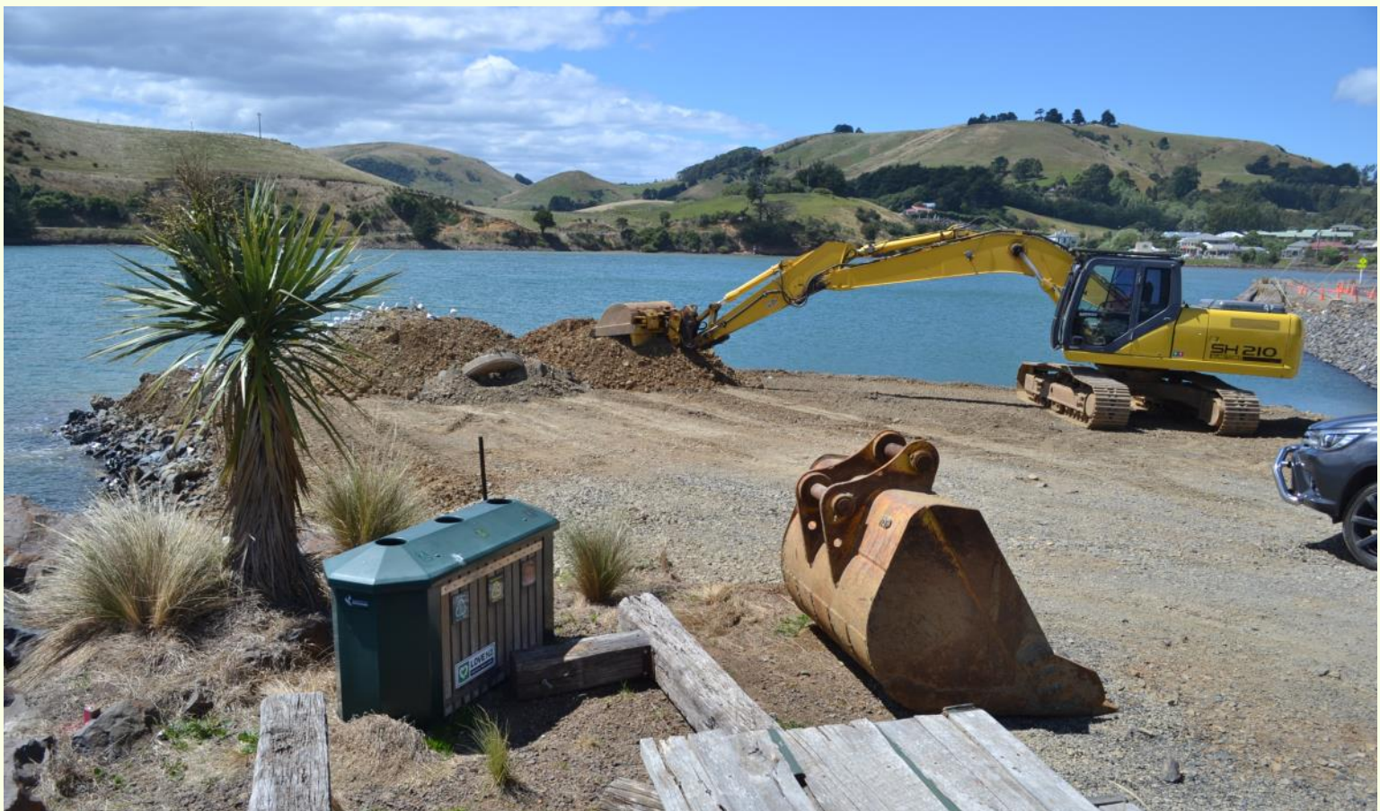
Progress continues at the jetty with more reclamation to make way for the new boatshed and ramp.
