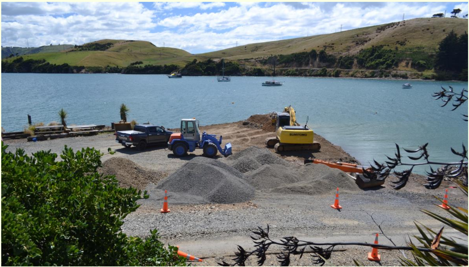
Progress continues at the jetty with more reclamation to make way for the new boatshed and ramp.
